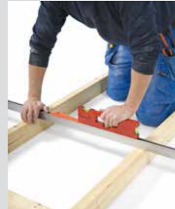
4. You can check inclines using the gradient wedge.
